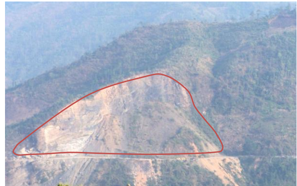
Plate 1. Landslide area at the outskirts of Saitual town
